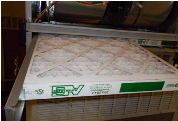
FIGURE 10 Install Left 2" Filter
