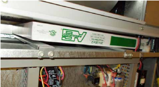
FIGURE 10 Install Left 2" Filter
