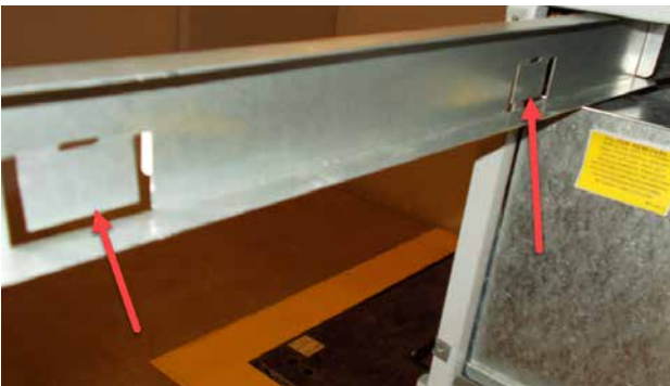
FIGURE 5 Bend Filter Tabs Down
