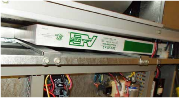
FIGURE 10 Install Left 2" Filter
