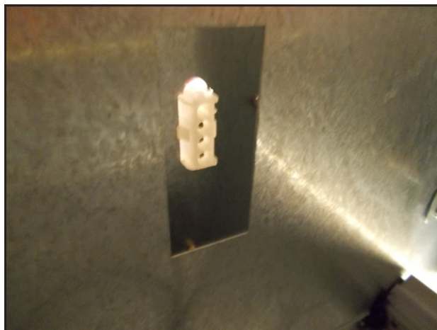
FIGURE 9 Control Plug Centered in Plug Access Opening
