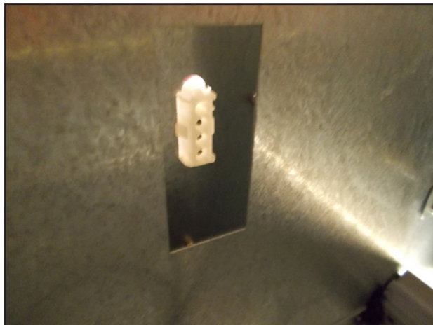
FIGURE 9 Control Plug Centered in Plug Access Opening
