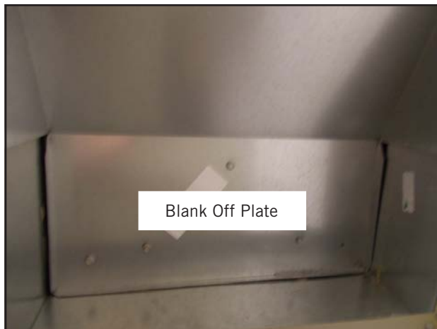
FIGURE 4 Remove Blank Off Plates (Both Sides)
