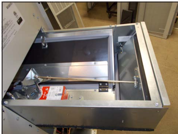
FIGURE 10 Install Economizer
