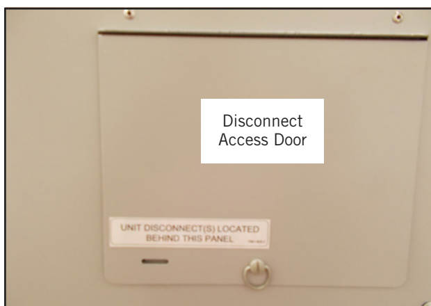
FIGURE 1 Disconnect Power
