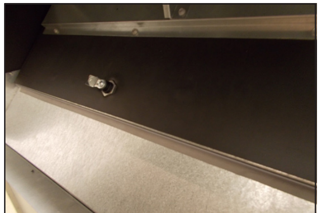
FIGURE 24 Exhaust Blade and Latch
