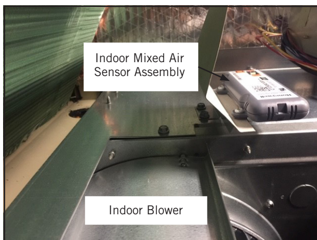
FIGURE 13 Install Indoor Mixed Air Sensor Assembly
