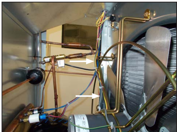
FIGURE 19 Route Wires and Secure with Ties
