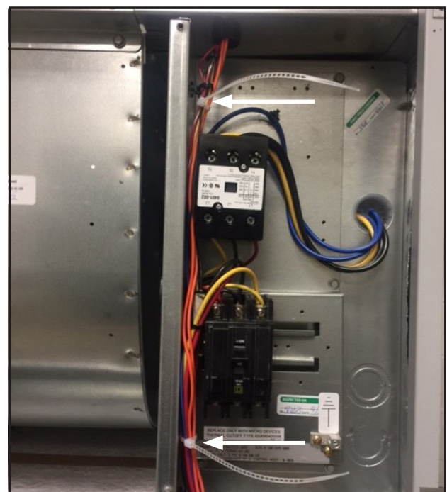
FIGURE 15 Secure Sensor Wires with Ladder Ties
