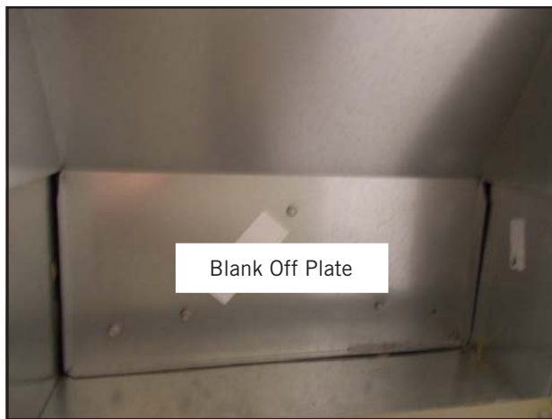
FIGURE 4 Remove Blank Off Plates (Both Sides)
