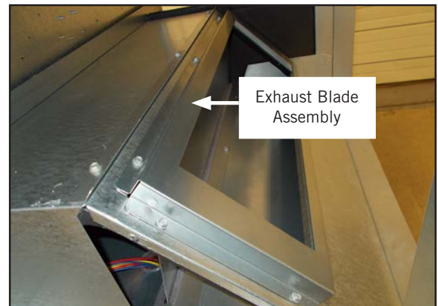
FIGURE 7 Install Exhaust Blade Assembly
