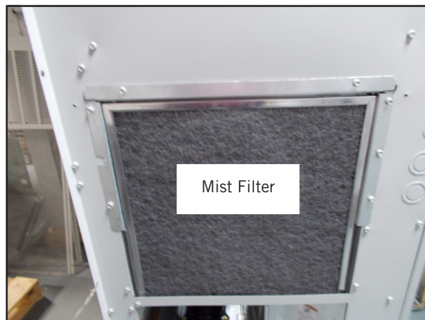
FIGURE 16 Install Mist Filters
