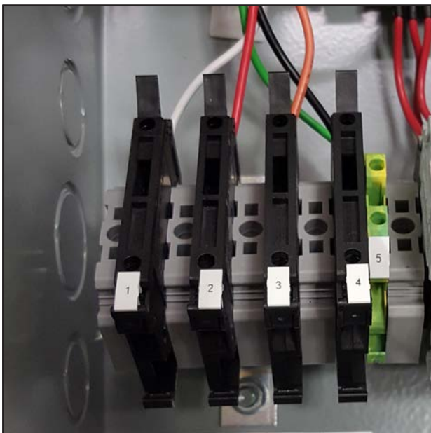
FIGURE 15 LC6000 Fused Power Supply Terminal
