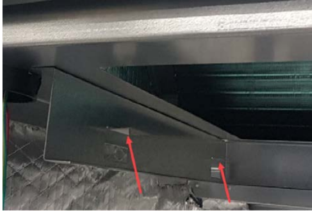
FIGURE 10 Bend Filter Tabs Down
