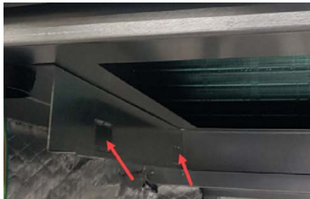
FIGURE 10 Bend Filter Tabs Down
