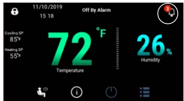
FIGURE 19 Active Alarms Displayed on Main Screen
