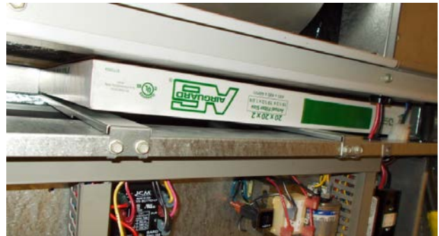
FIGURE 42 Install Left 2" Filter
