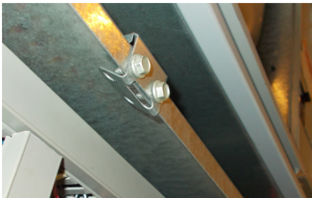
FIGURE 40 Re-Install Screws and Bend Tabs Up
