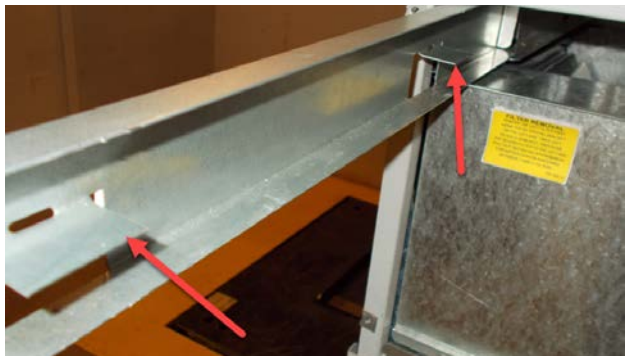
FIGURE 36 Filter Tabs in Up Position
