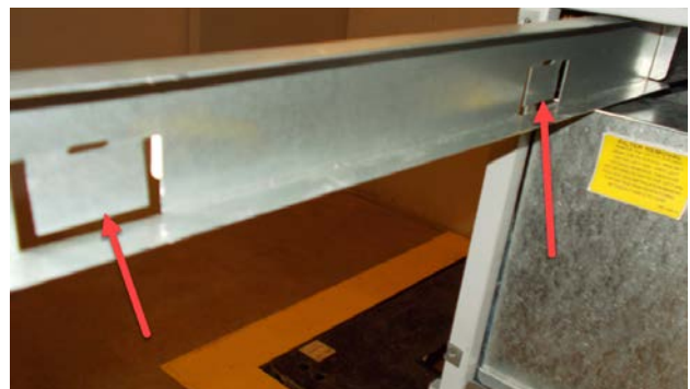
FIGURE 37 Bend Filter Tabs Down
