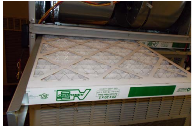
FIGURE 42 Install Left 2" Filter
