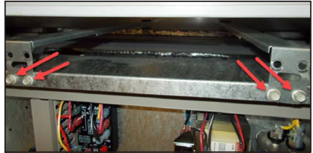
FIGURE 6 Remove Four Screws
