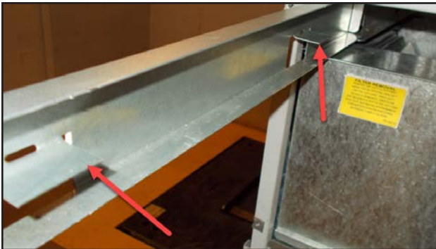
FIGURE 4 Filter Tabs in Up Position
