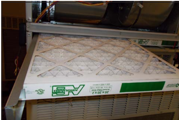
FIGURE 10 Install Left 2" Filter
