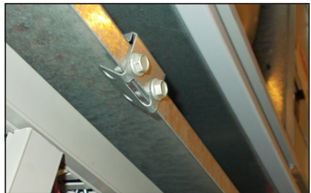
FIGURE 8 Re-Install Screws and Bend Tabs Up
