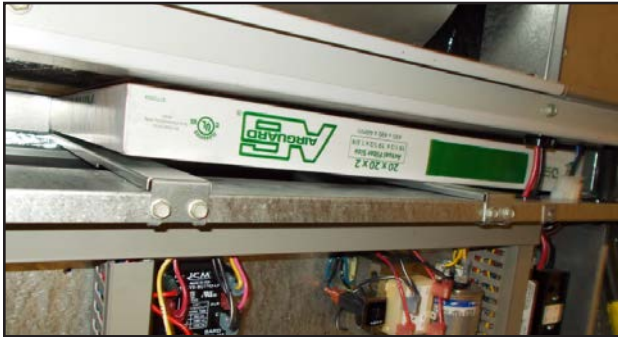
FIGURE 10 Install Left 2" Filter
