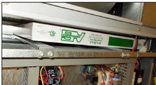
FIGURE 10 Install Left 2" Filter
