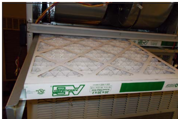
FIGURE 10 Install Left 2" Filter
