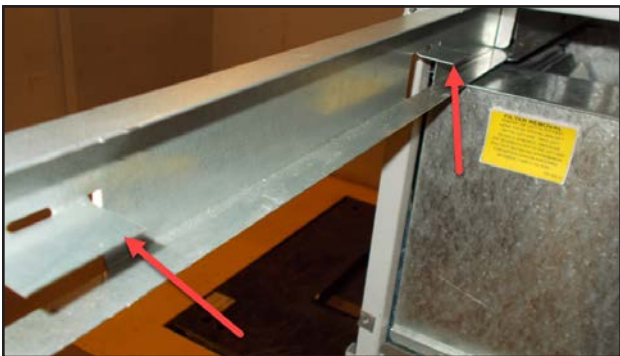
FIGURE 4 Filter Tabs in Up Position
