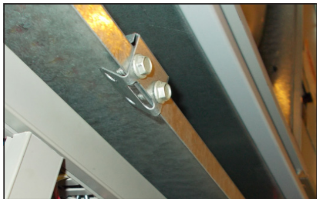
FIGURE 8 Re-Install Screws and Bend Tabs Up
