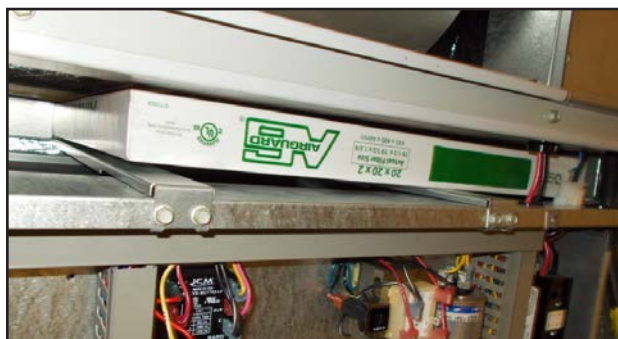
FIGURE 10 Install Left 2" Filter
