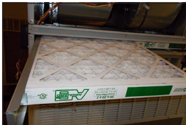
FIGURE 10 Install Left 2" Filter
