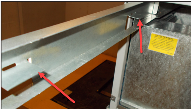
FIGURE 4 Filter Tabs in Up Position
