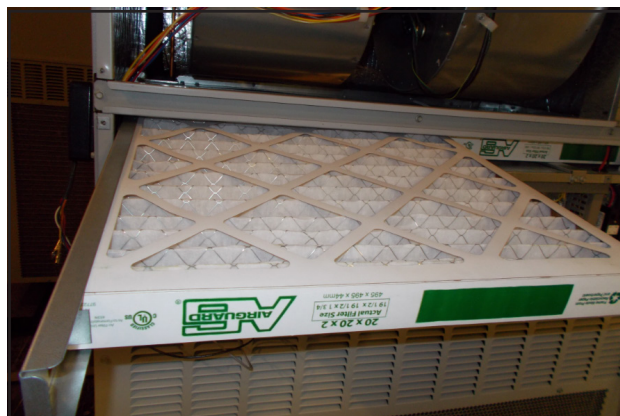
FIGURE 10 Install Left 2" Filter
