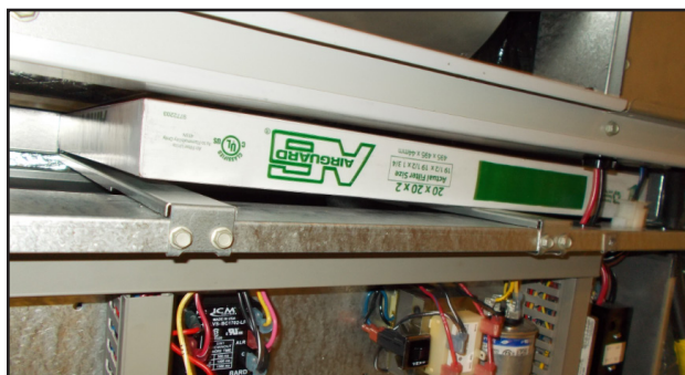
FIGURE 10 Install Left 2" Filter
