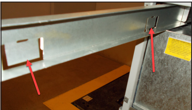
FIGURE 5 Bend Filter Tabs Down
