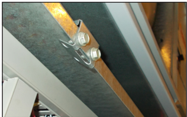
FIGURE 8 Re-Install Screws and Bend Tabs Up
