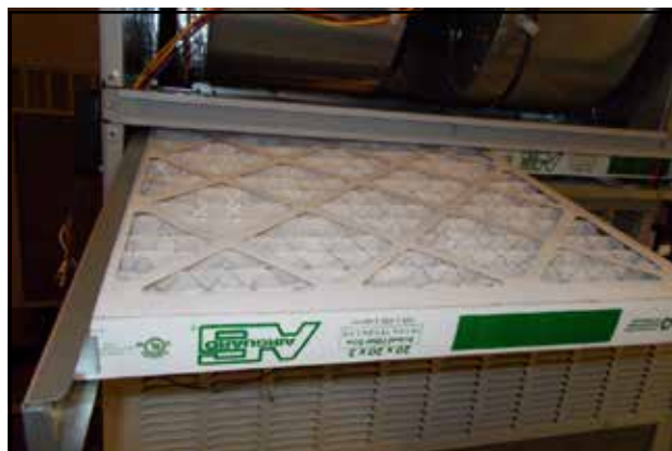
FIGURE 10 Install Left 2" Filter
