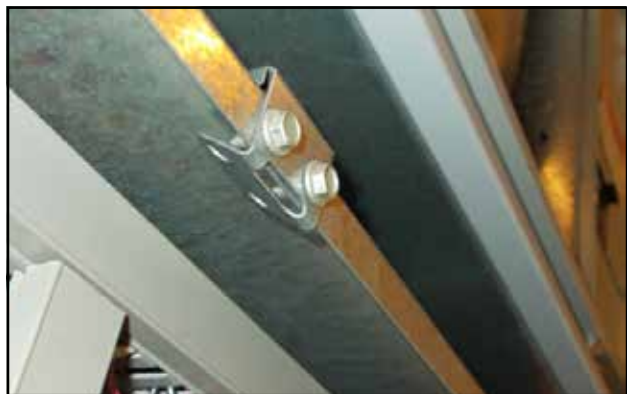
FIGURE 8 Re-Install Screws and Bend Tabs Up
