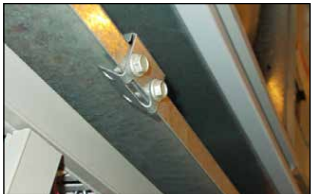
FIGURE 8 Re-Install Screws and Bend Tabs Up
