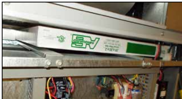
FIGURE 10 Install Left 2" Filter
