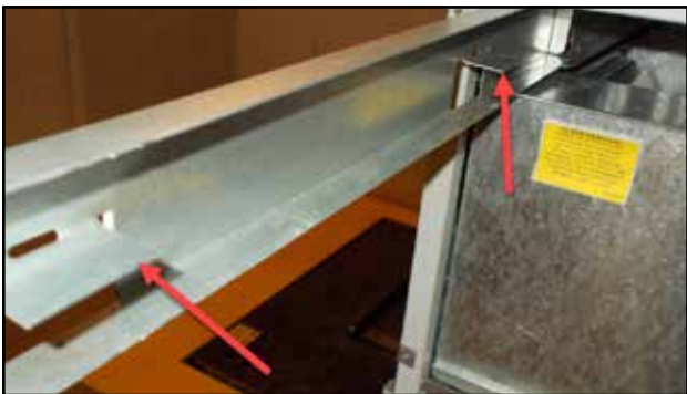
FIGURE 4 Filter Tabs in Up Position
