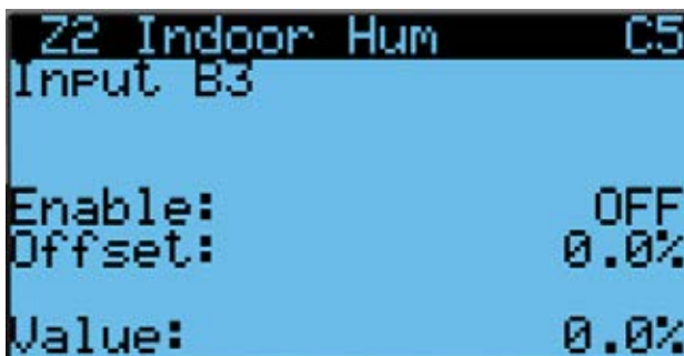
FIGURE 37 Enable/Disable Zone 2 Indoor Humidity Sensor
