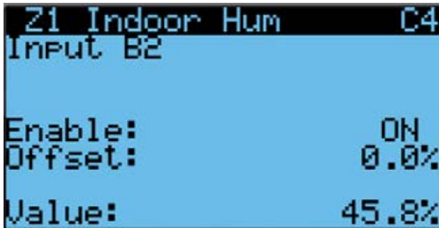
FIGURE 36 Enable/Disable Zone 1 Indoor Humidity Sensor
