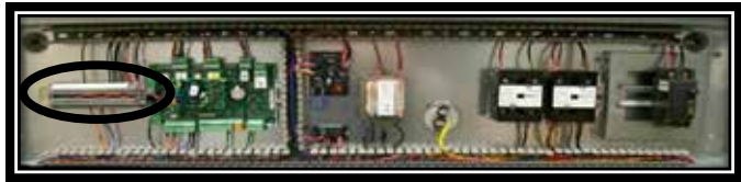
FIGURE 29 Communication Wiring: Termination at the First Wall-Mount Unit
