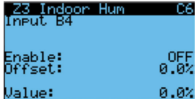
FIGURE 46 Enable/Disable Zone 3 Indoor Humidity Sensor
