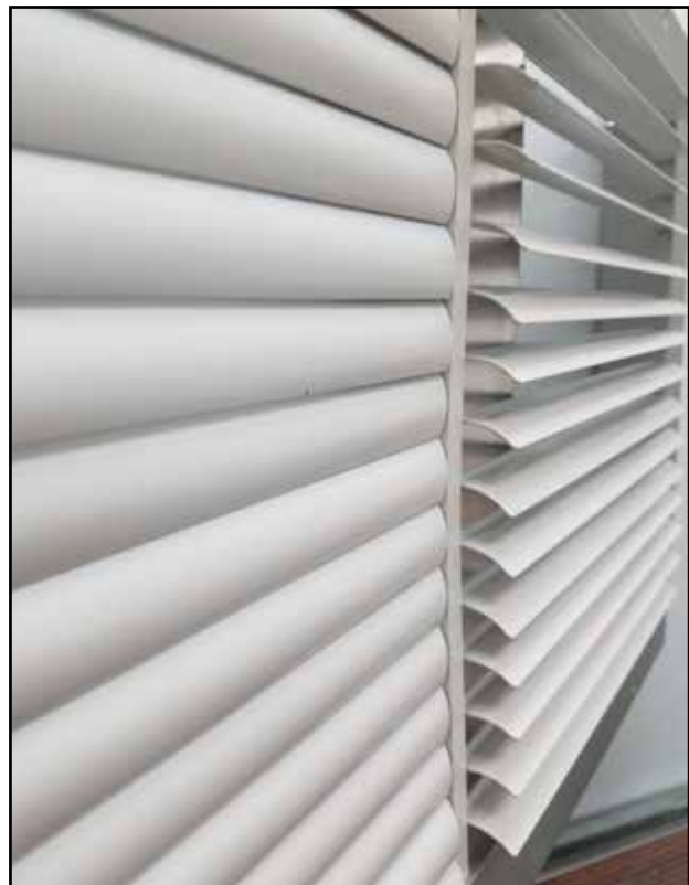
Diverter blades as shipped (left), and after raising (right)
