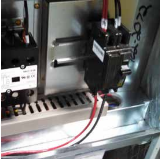
FIGURE 13 Wire Routing
