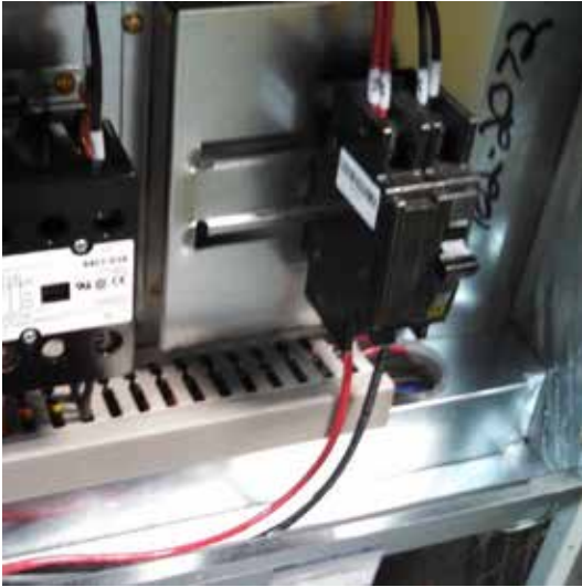
FIGURE 16 Side Communication and Power Wire Entrances (Recommended)
