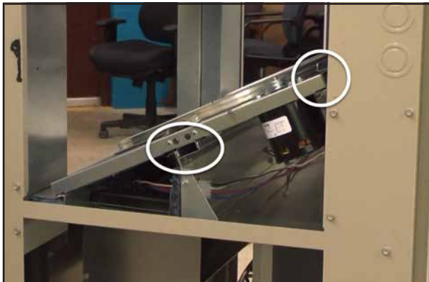
FIGURE 31 Cassettes Installed Properly into Cassette Rack and Cassette Mounting Rail
