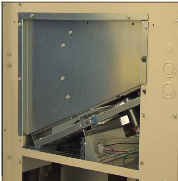
FIGURE 43 Install Upper Side Covers
