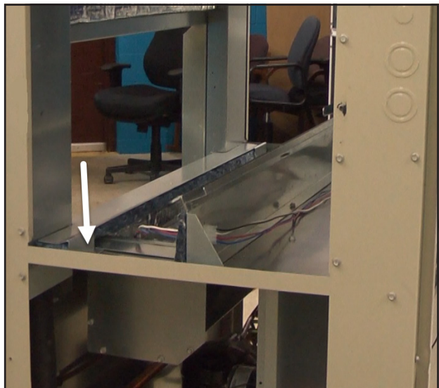
FIGURE 29 Install Additional Screws into Rear ERV Mounting Rail
