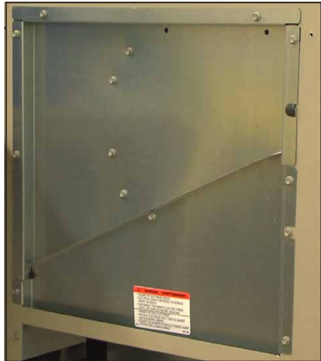
FIGURE 44 Install Lower Side Covers
