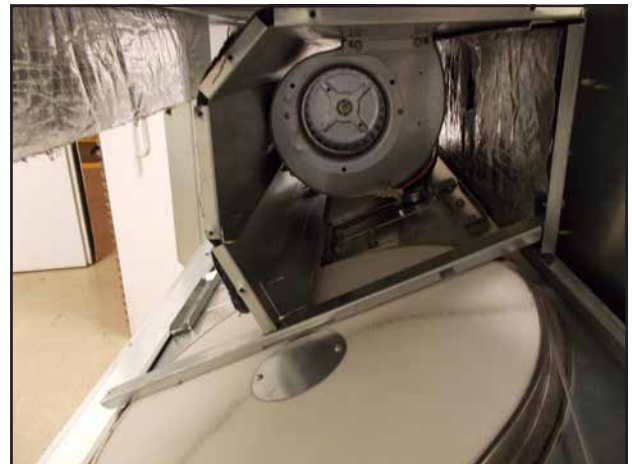
FIGURE 33 Upper Blower Assembly Over Cassettes
