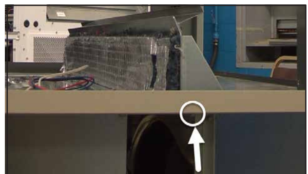
FIGURE 17 Insert Screws Through Condenser Section into Center Cassette Rack
