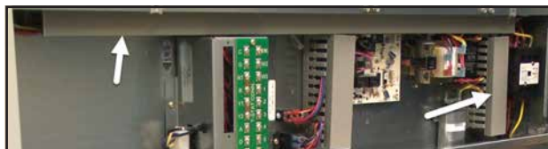
FIGURE 23 Remove Two Wire Channel Covers
