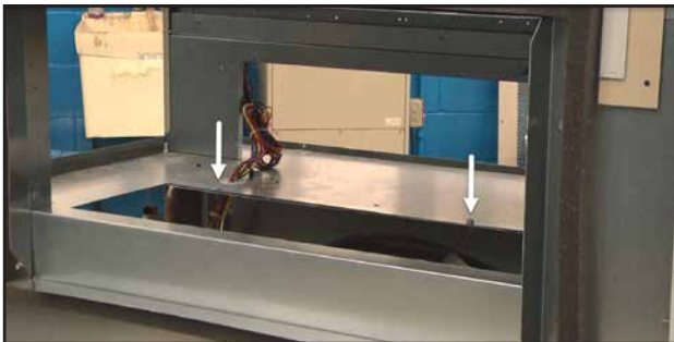
FIGURE 13 Install Exhaust Blower Base
