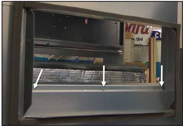
FIGURE 28 Install Rear ERV Mounting Rail
