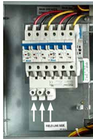
FIGURE 10 VAC Supply Wiring Landing Points
