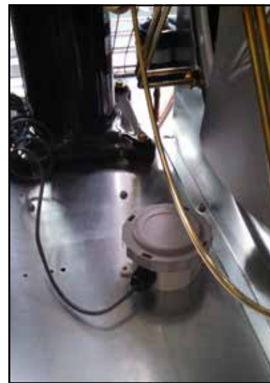
FIGURE 3 Outdoor Sensor Installation
