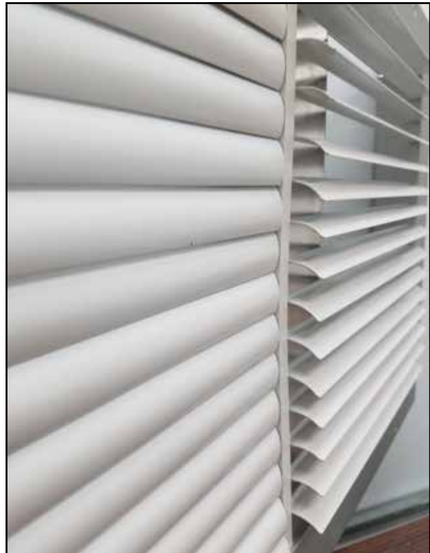
FIGURE 6 Downward Curved Diverter Blades
