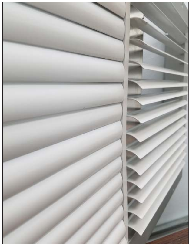
FIGURE 6 Downward Curved Diverter Blades
