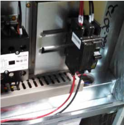
FIGURE 14 Wire Routing
