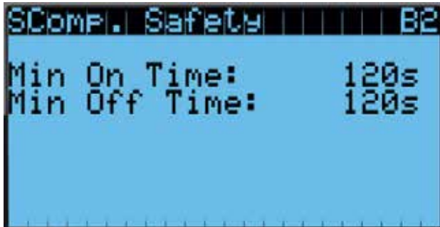
FIGURE 32 Adjusting Compressor Delays
