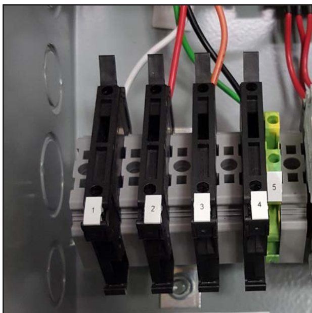
FIGURE 2 LC6000 Fused Power Supply Terminals
