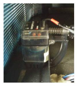
FIGURE 35 Outdoor Condensate Sensor
