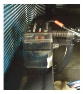
FIGURE 35 Outdoor Condensate Sensor
