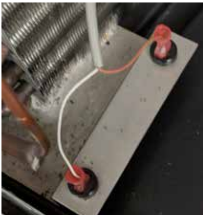
FIGURE 35 Outdoor Condensate Sensor
