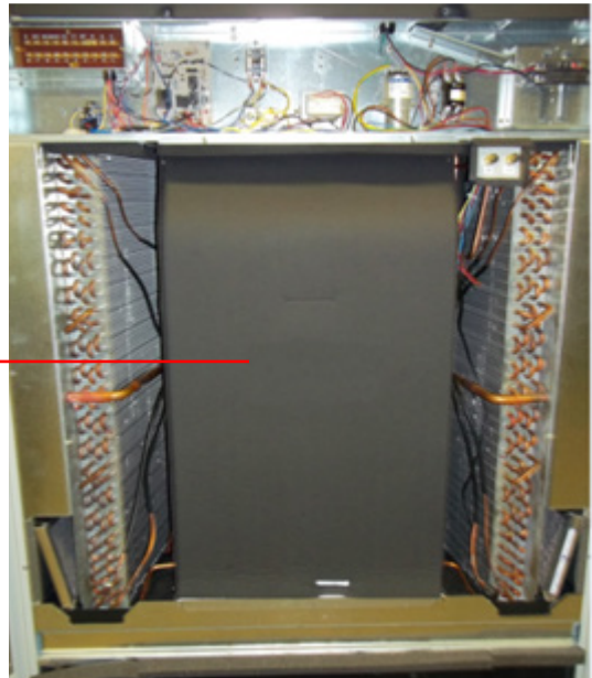
FIGURE 4 Removal of Air Duct
