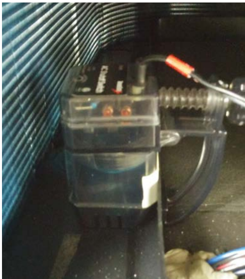
FIGURE 19 Outdoor Condensate Sensor
