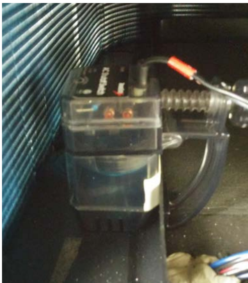
FIGURE 19 Outdoor Condensate Sensor
