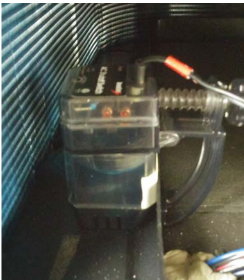
FIGURE 19 Outdoor Condensate Sensor
