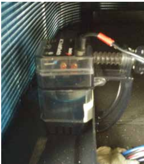
FIGURE 19 Outdoor Condensate Sensor
