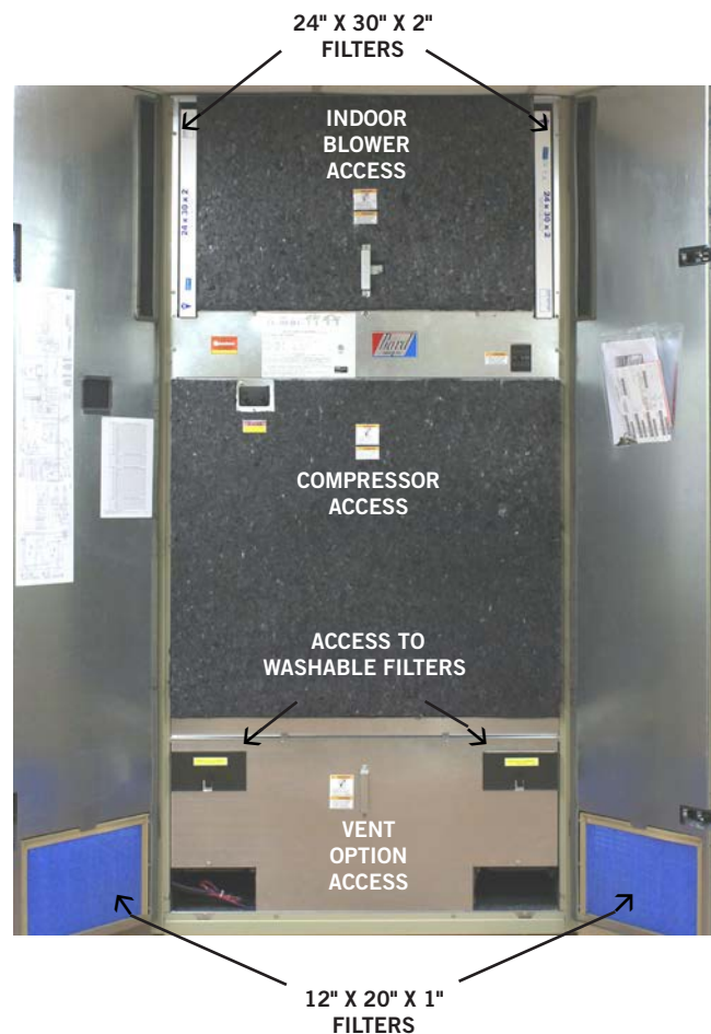
FIGURE 9 Filter Location
