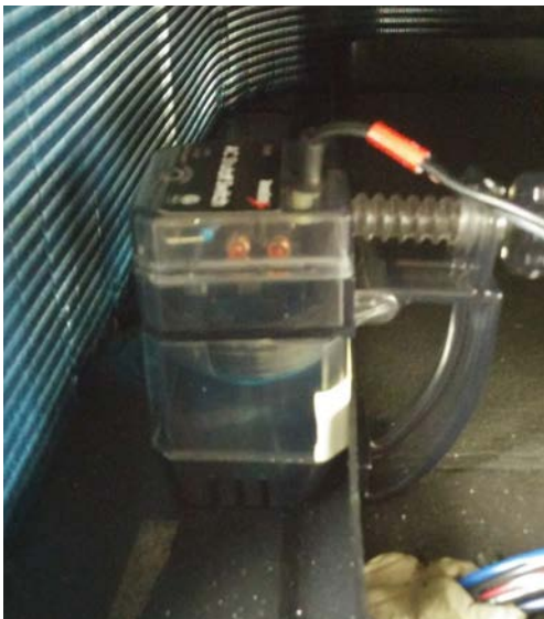
FIGURE 35 Outdoor Condensate Sensor
