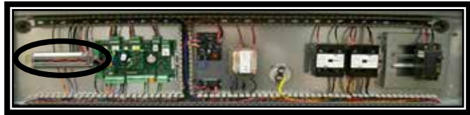
FIGURE 25 Communication Wiring: Termination at the First Wall-Mount Unit
