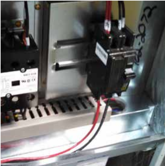
FIGURE 13 Wire Routing
