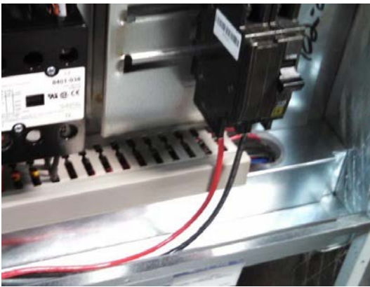
FIGURE 16 Side Communication and Power Wire Entrances (Recommended)
