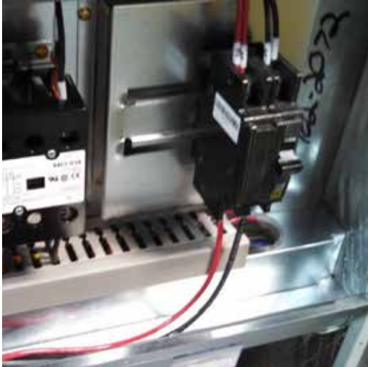
FIGURE 13 Wire Routing
