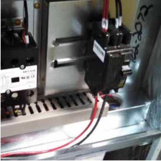
FIGURE 13 Wire Routing
