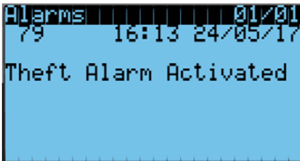
FIGURE 5 LV1000 Anti-Theft Alarm Screen
