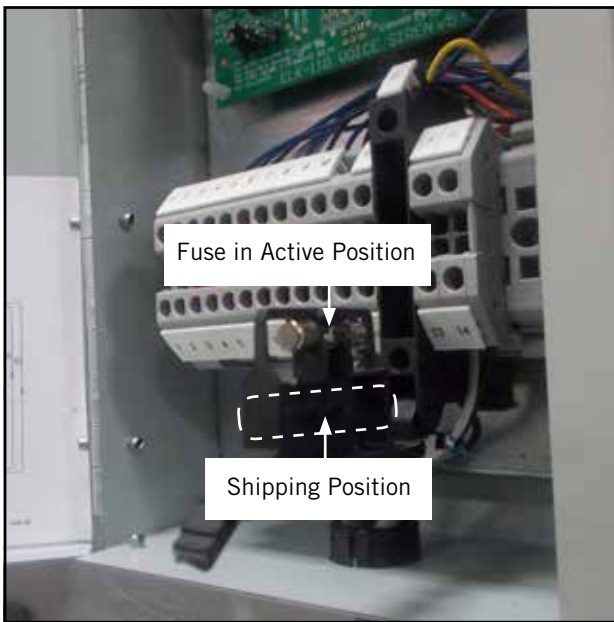
FIGURE 1 BG1000 Fused Power Supply Terminal
