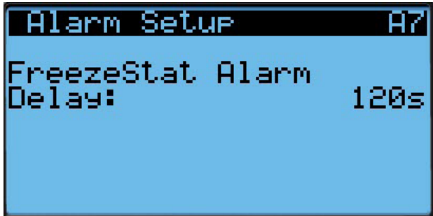
FIGURE 21 Adjusting Freezestat Alarm Delay
