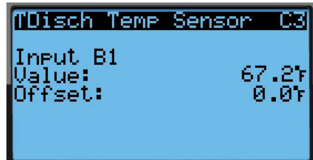
FIGURE 25 Adjusting Discharge Temperature Input
