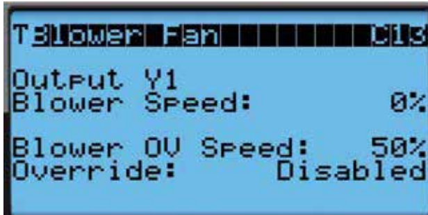
FIGURE 17 Putting Blower Output into Override Mode
