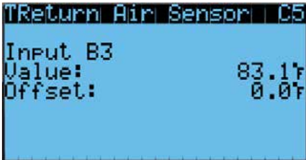
FIGURE 6 Adjusting Return Air Sensor
