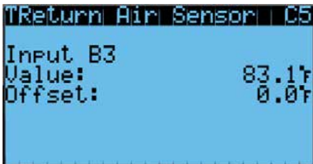
FIGURE 6 Adjusting Return Air Sensor
