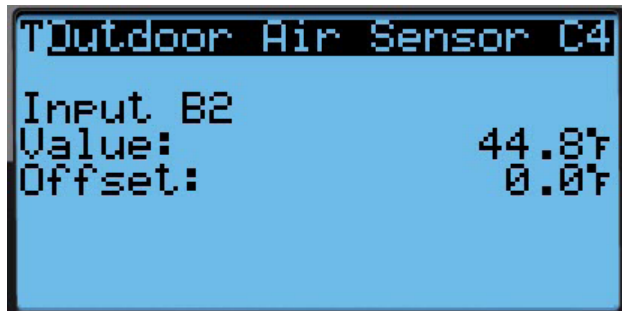
FIGURE 37 Outdoor Air Sensor
