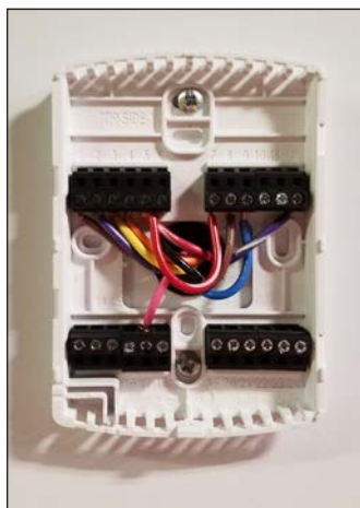
FIGURE 4 Connect Wires to Thermostat Sub-Base
