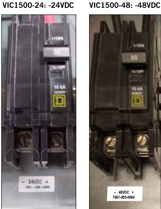
FIGURE 2 VIC1500 Connection Points: Power Supply
