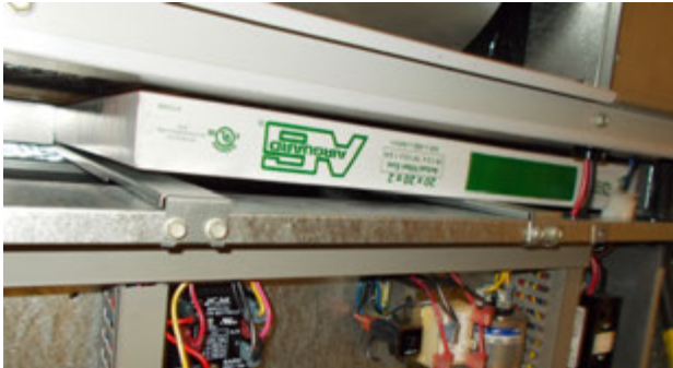
FIGURE 10 Install Left 2" Filter
