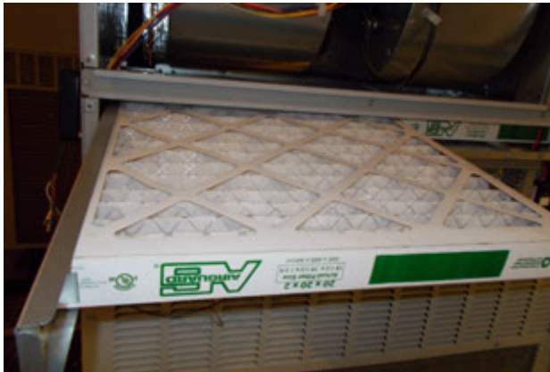
FIGURE 10 Install Left 2" Filter
