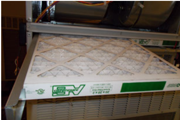
FIGURE 10 Install Left 2" Filter
