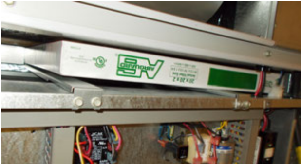
FIGURE 10 Install Left 2" Filter
