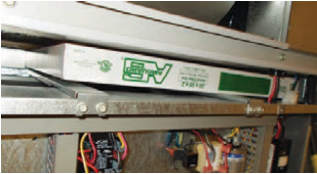
FIGURE 10 Install Left 2" Filter
