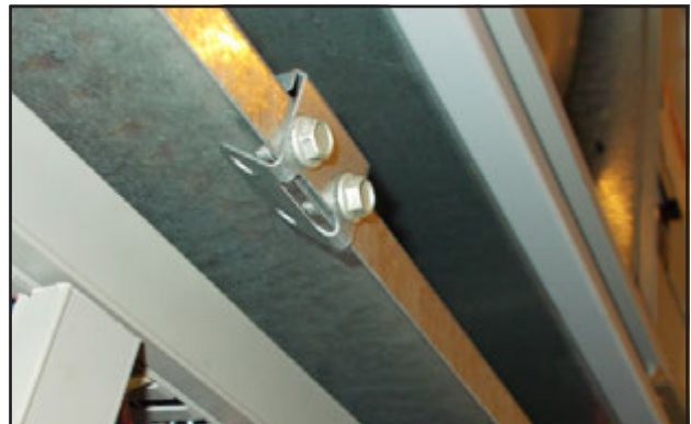
FIGURE 65 Re-Install Screws and Bend Tabs Up
