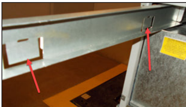
FIGURE 62 Bend Filter Tabs Down
