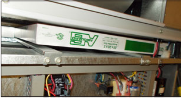
FIGURE 66 Install Right 2" Filter
