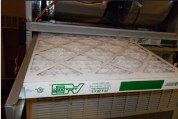
FIGURE 67 Install Left 2" Filter
