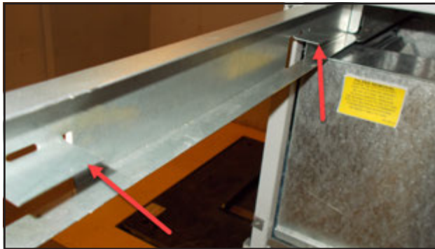
FIGURE 61 Filter Tabs in Up Position
